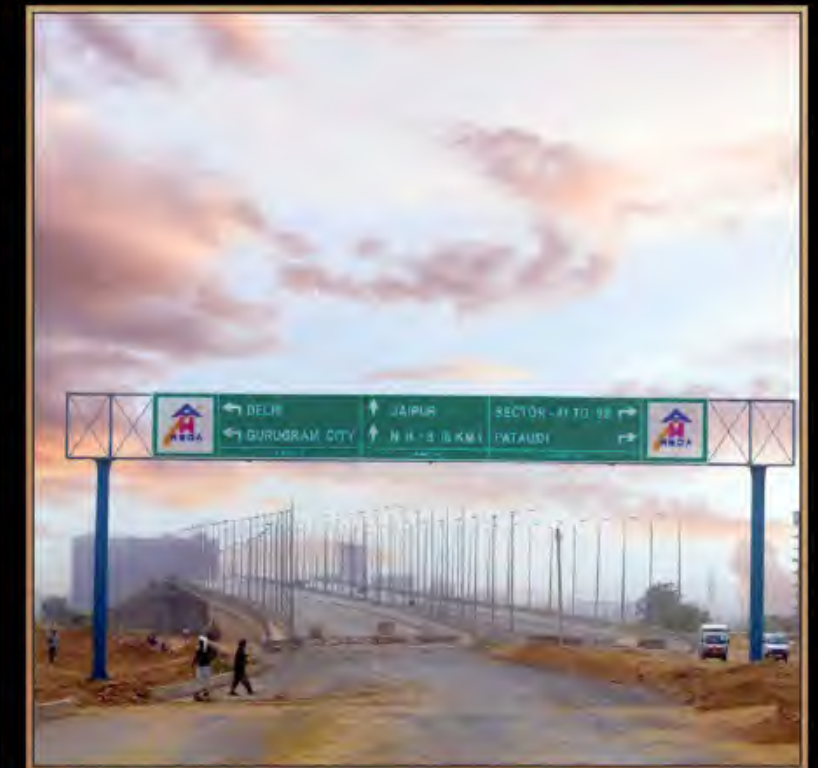
Rail Over Bridge (ROB): As part of the Dwarka Expressway, this 1300-meter, six-lane ROB has been developed to enhance connectivity.
